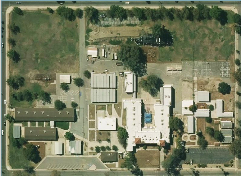
2014 Prior to Deconstruction
